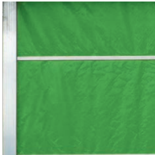
Ⓐ Stiffening bars inserted into form
